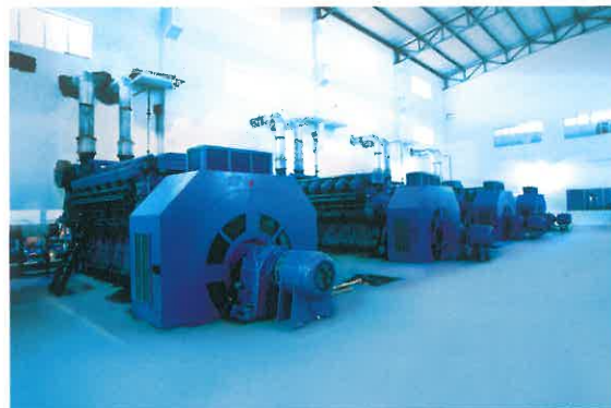
某大型集团发电机房采用我司2000kW×8重油发电机组群 The installation with the group of 2000kW× 8 HFO diesel generating sets from Guangzhou Diesel Engine Factory Co.,Ltd.
