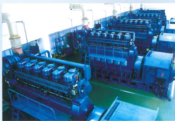
某大型企业发电机房采用我司1000kW×5重油发电机组群 The installation with the group of 1000kW× 5HFO diesel generating sets from Guangzhou Diesel Engine Factory Co.,Ltd.
