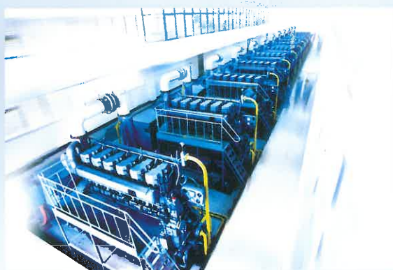
某大型家电企业发电机房采用我司500kW×12柴油发电机组群 The installation with the group of 500kW×12 diesel generating sets from Guangzhou Diesel Engine Factory Co.,Ltd.
